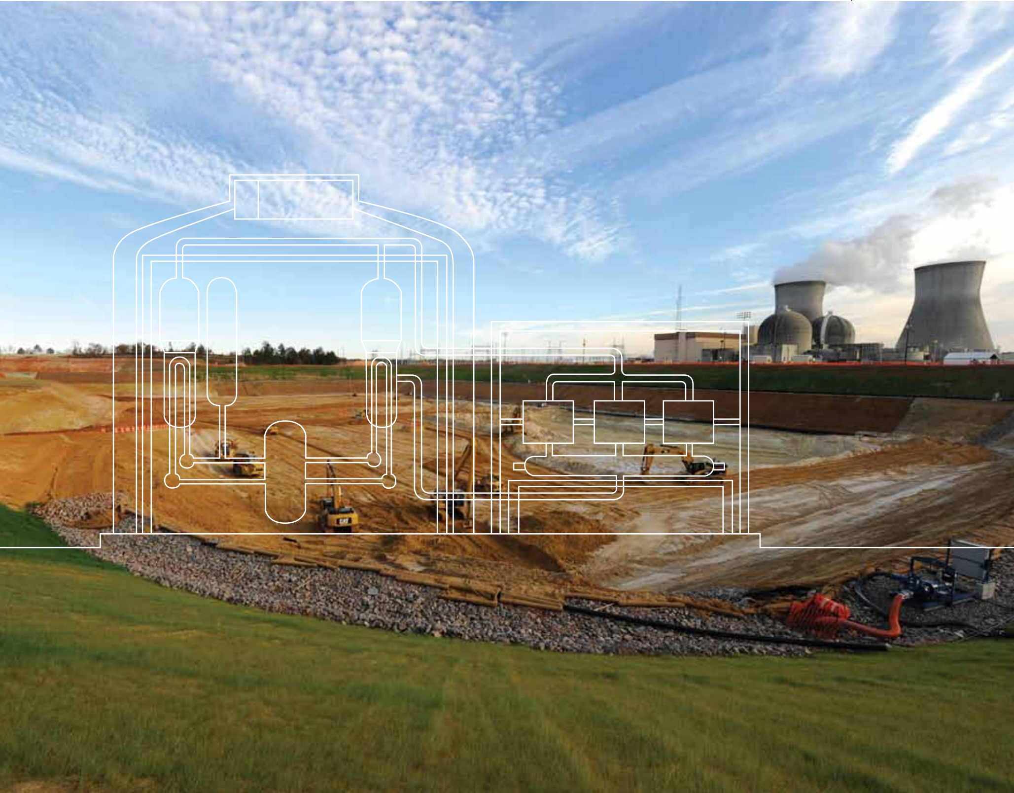
Operation excavation—Plant Vogtle construction: units 3 and 4, with the outline of a Westinghouse AP1000.
